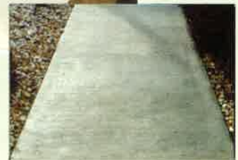
Micro-Crete can be trowelled smooth or broomed for a greater non-skid surface
